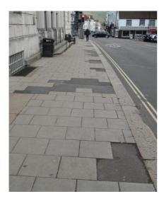
The possibility of having bollards to prevent pavement parking has been suggested but that would probably cause more traffic congestion Essentially the problem is due to the sub-base below the slabs not being strong enough to withstand the weight of lorries. Whilst this could be remedied it is expensive and more details of costs are being sought.
